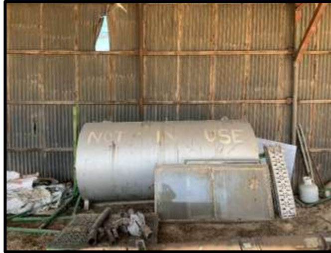
Image 2: One of the ASTs found in the shed near the residential dwelling onsite. Other notable materials found in this shed include a gas bottle, farming equipment, pesticides and herbicides.
