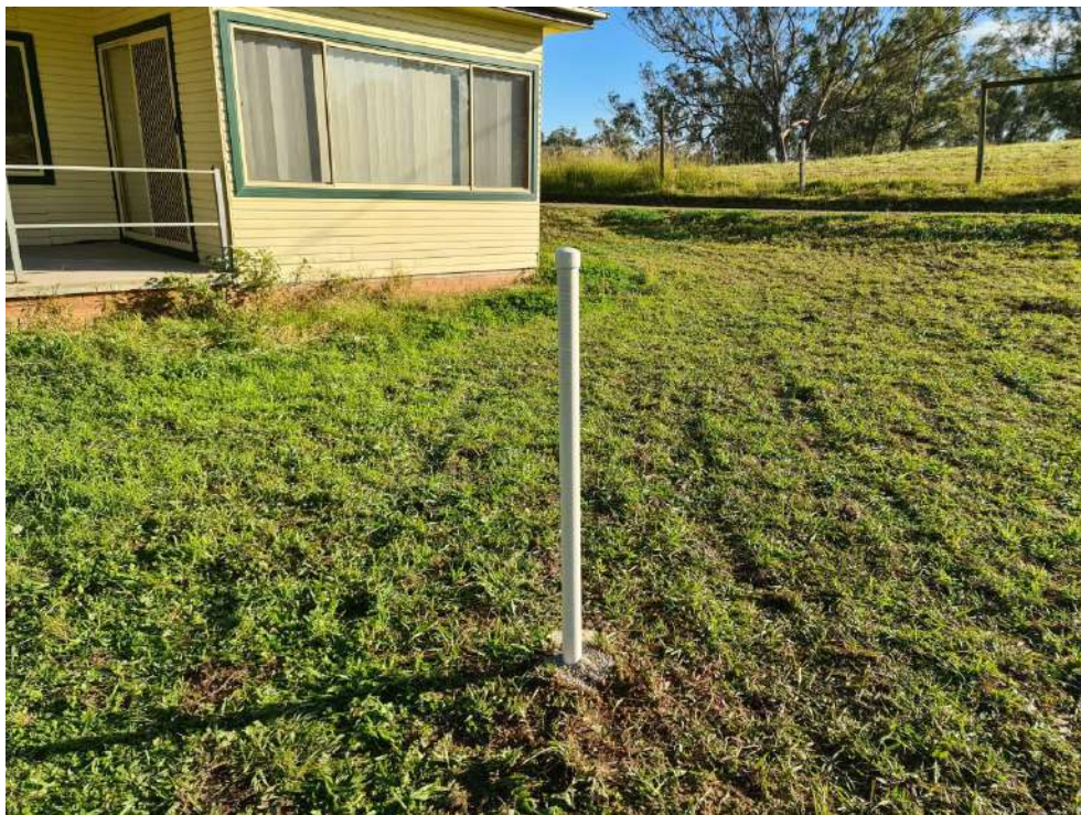
Photograph 3: 50 mm PVC riser of a newly constructed well. Looking northwest
