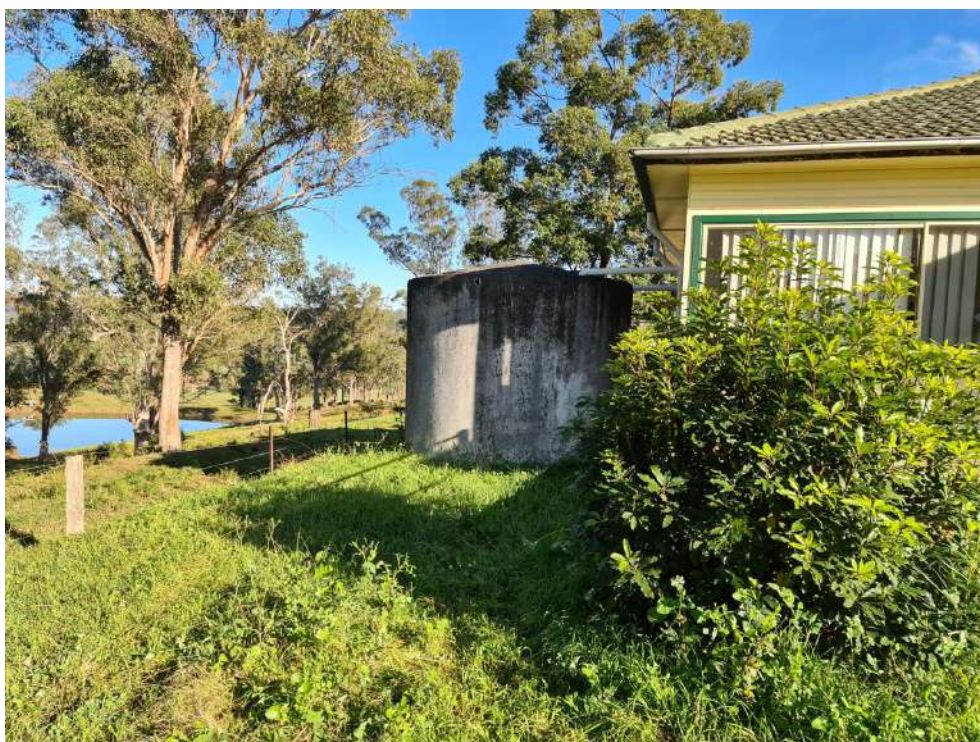
Photograph 4: Rainwater tanks at main building. Looking south.
