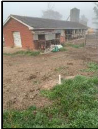
Image 4: In the foreground that water monitoring well identified as Well 1. This image depicts the dairy shed onsite, looking north-east. Behind this building the silos can be seen also. Following these properties the site slopes downwards towards the Nepean River.
