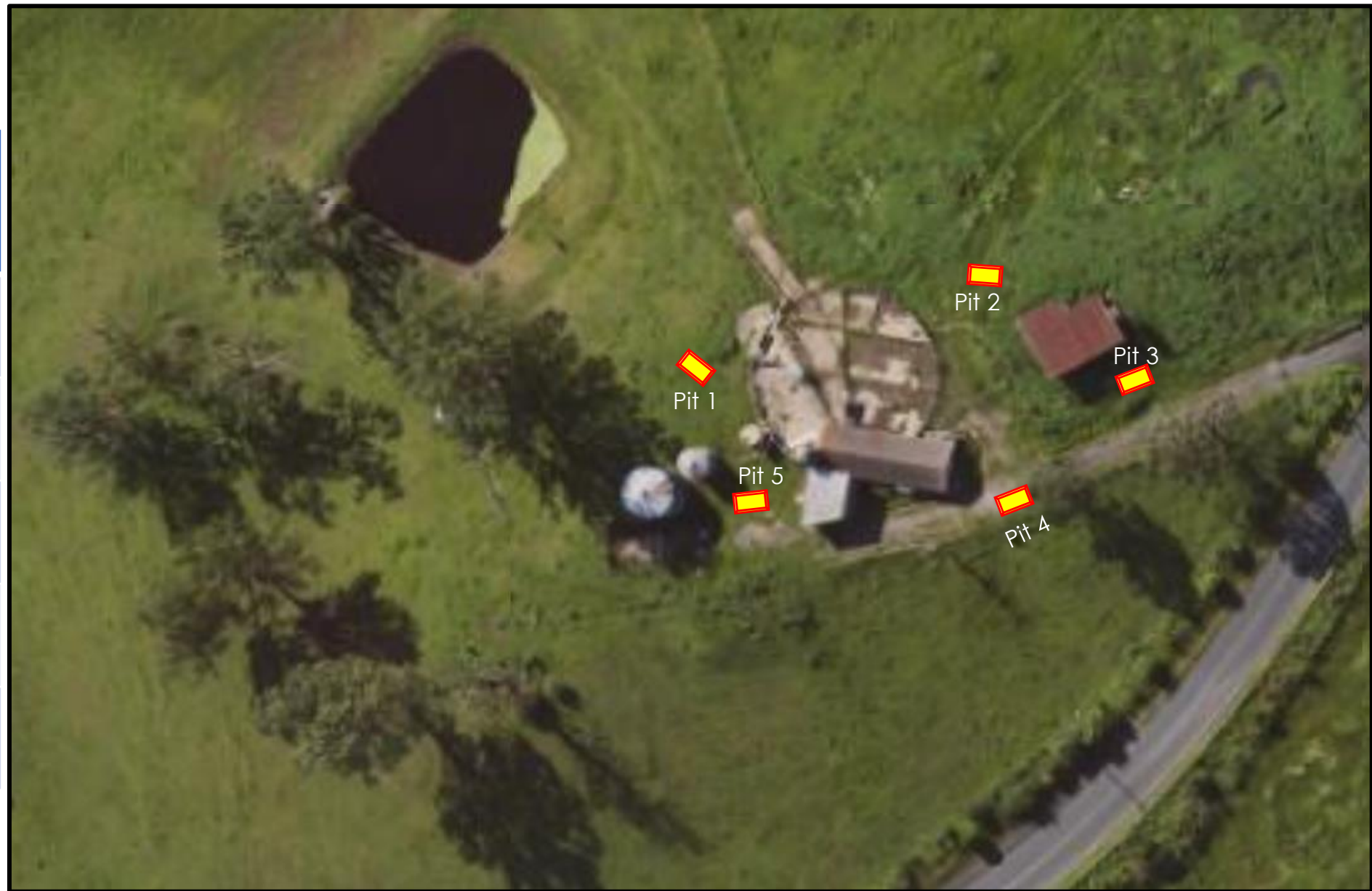
Figure 10 Pit Locations 1-5 (proximal to silos and southern shed) Project 1290 Greendale Road, Wallacia, NSW, 2745
