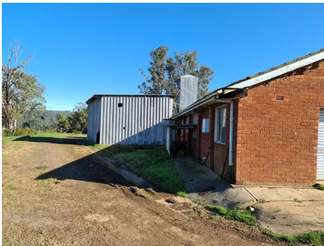
Photograph 28: Brick and metal diary sheds. Looking south.
