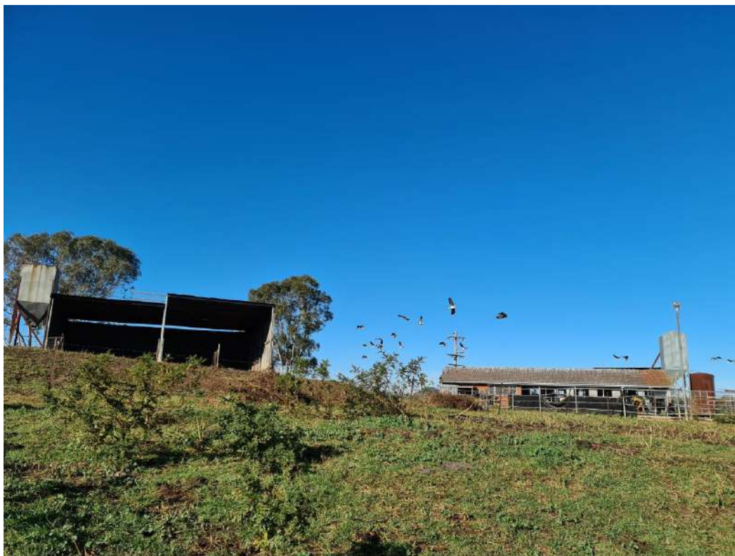
Photograph 21: Dairy shed (right) and agricultural shed. Looking south.
