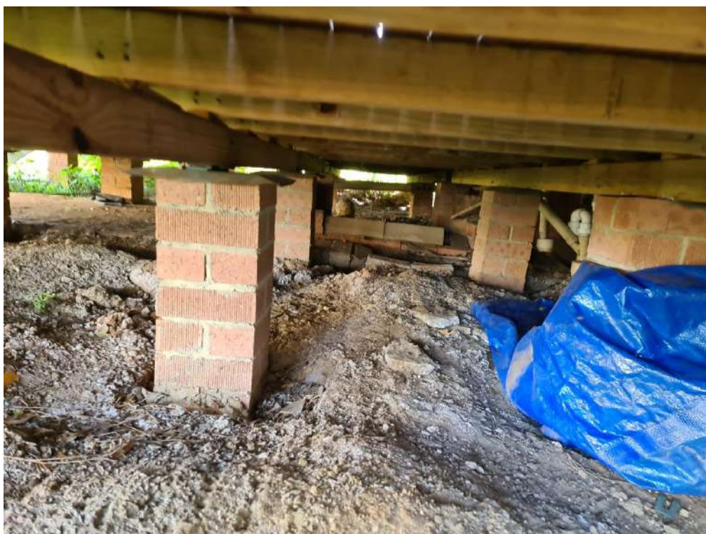
Photograph 6: Main House. Crawl space.
