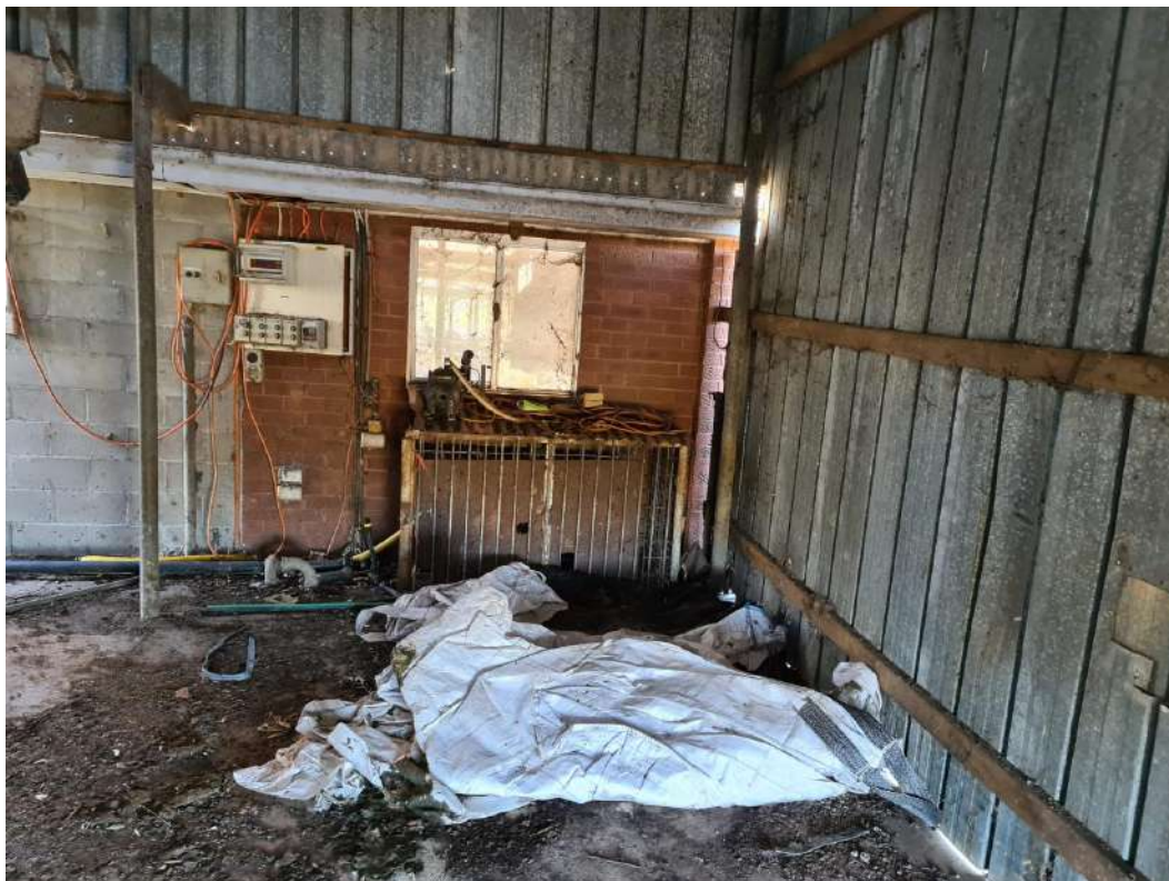
Photograph 29: Interior of brick shed. Disused pump equipment in cage.
