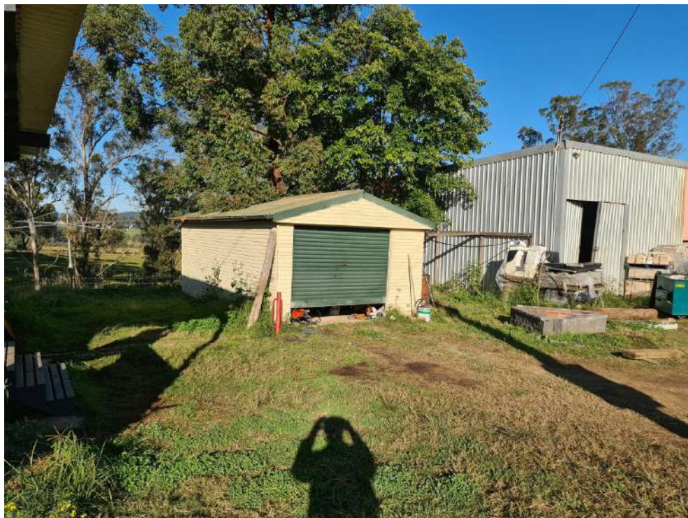
Photograph 7: View of garage and sheds west of homestead. Looking south.
