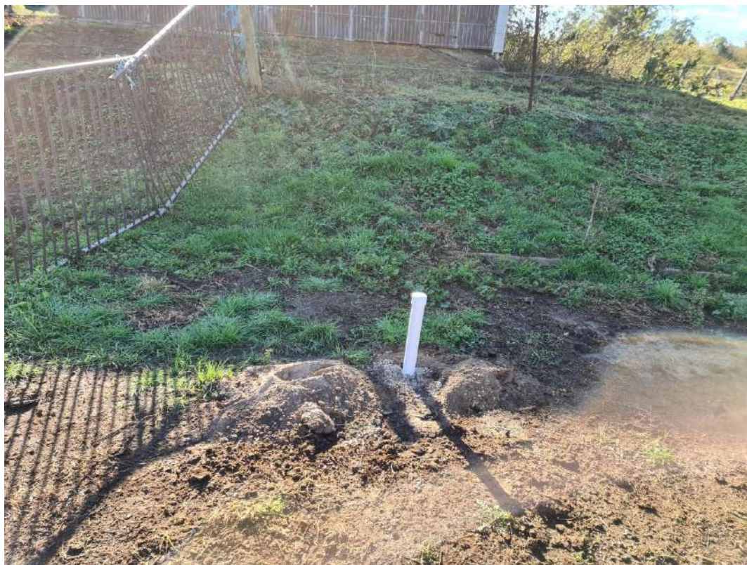
Photograph 27: 50 mm PVC riser of newly constructed groundwater monitoring well.
