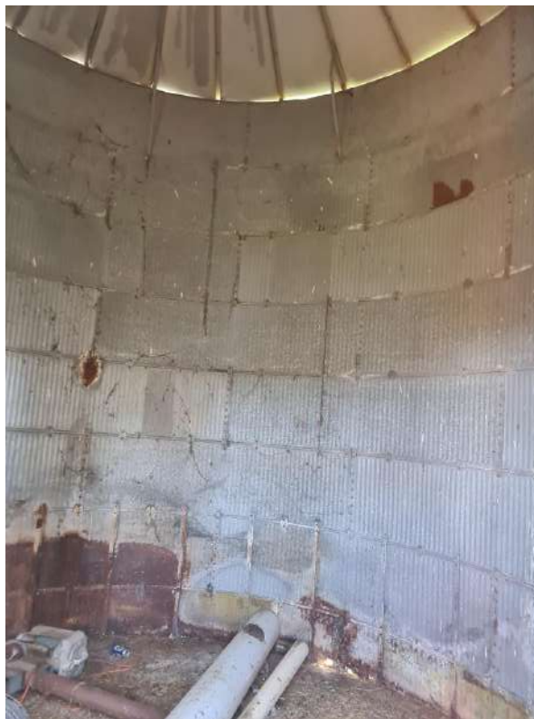
Photograph 31: Interior of disused silo.
